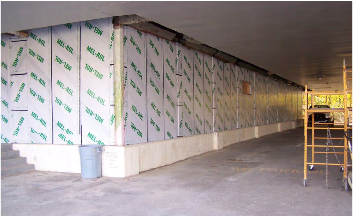
A structurally unsound cinderblock wall at the Boys and Girls Club has been replaced with a reinforced flood resistant wall.
