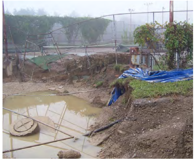
Temporary flood measures were breached along Watson Blvd.
