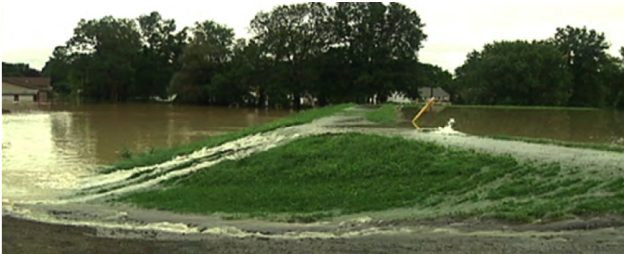
Backwater effect flooding caused overtopping of the levee around Fairmont Park in several locations.
