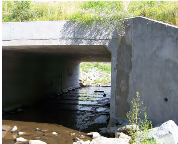
New box culvert at Struble Road.
