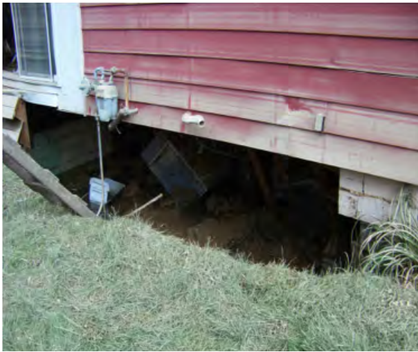
Flood waters undermined foundations in several neighborhoods.
