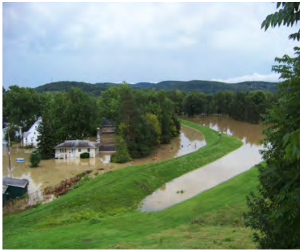
Backwater flooding led to overtopping of levee around Fairmont Park.
